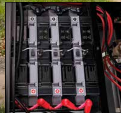
Batteries require no daily maintenance.
